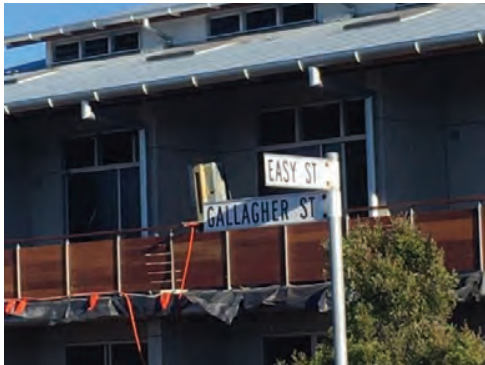
Stage 5 is located partly at the corner of Easy Street and Gallagher Street. This photo shows part of the recently completed pocket living development (now known as "Easy Street Living").
